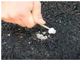
Remove cap for anchor access
