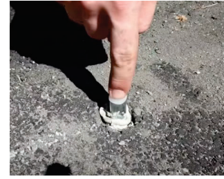
Insert Metal Sleeve
