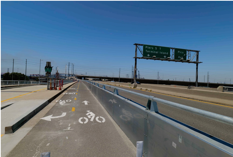
Smooth backside for safe bicycle passage
