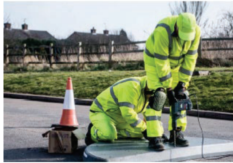
4. Anchor in place
