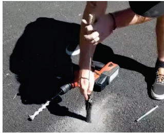
Wire brush hole to remove drill powder from cavity
