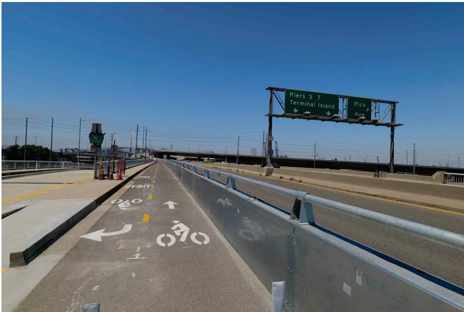
Smooth backside for safe bicycle passage
