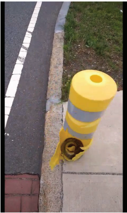
Damaged K71 posts remaining upright.
