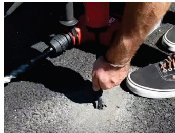
Blow out debris with air
